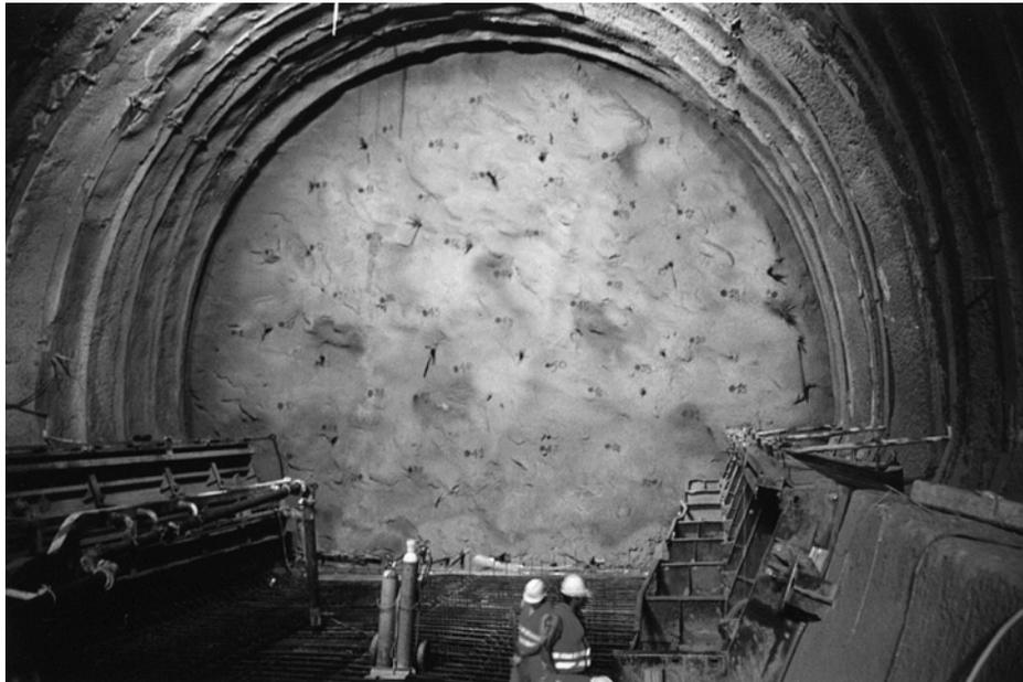
Fig. 1 – Raticosa tunnel, Italy: tunnel face supported by a temporary shotcrete shell and fiber-glass dowels.
